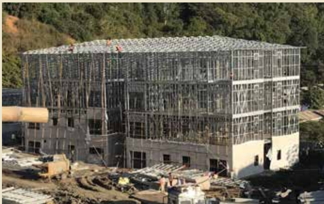
LGSF structure of building block
