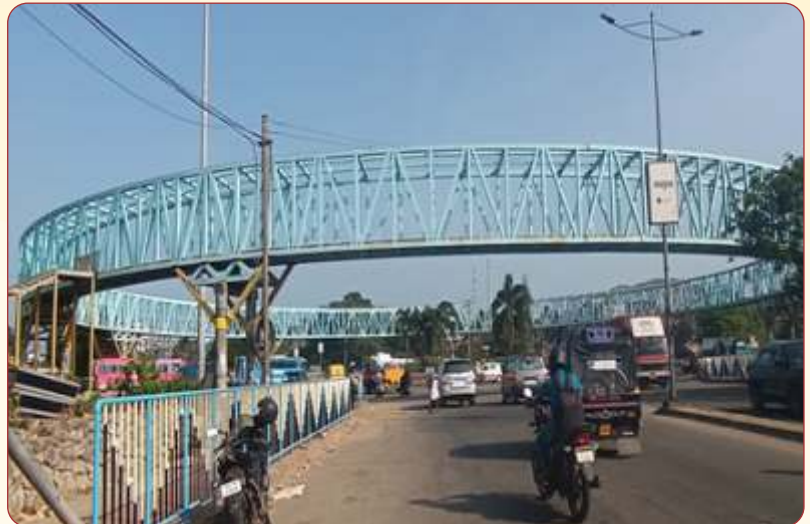
Roundabout after installation of Sky Walk
