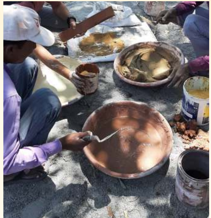
Use of traditional building materials
