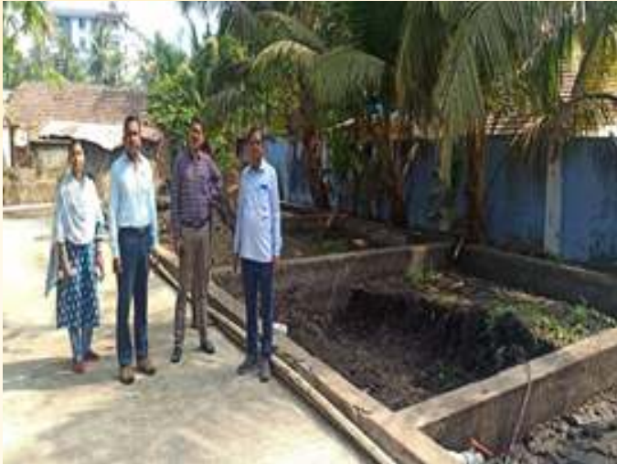
Sludge Drying Beds ( Sludge taken for Composting) STP View
