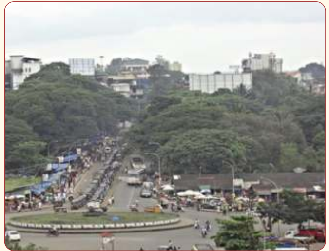
Roundabout before installation of Sky Walk
