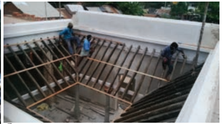
East side courtyard during restoration
