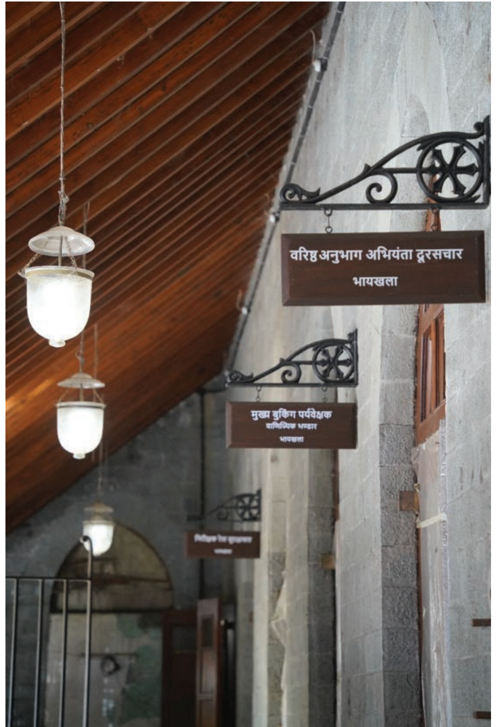
The original exposed basalt stone façade that was covered with layers of paint was revealed during the restoration process. Historic handi lights installed in the verandah
