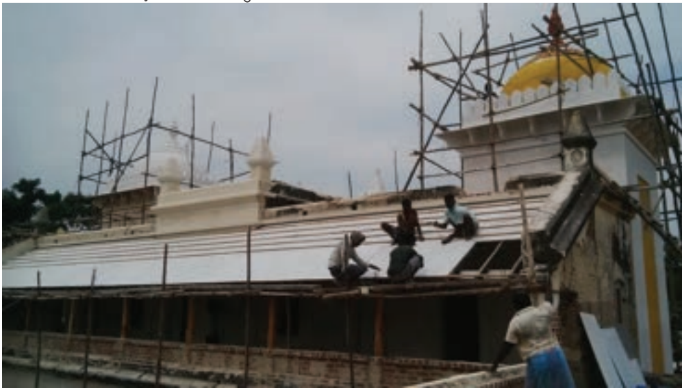
First floor corridor during restoration
