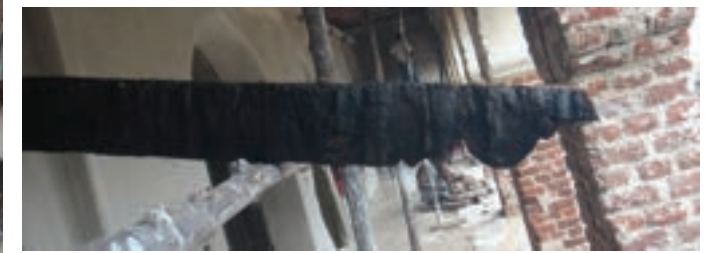
Palm rafters for central courtyard corridor
