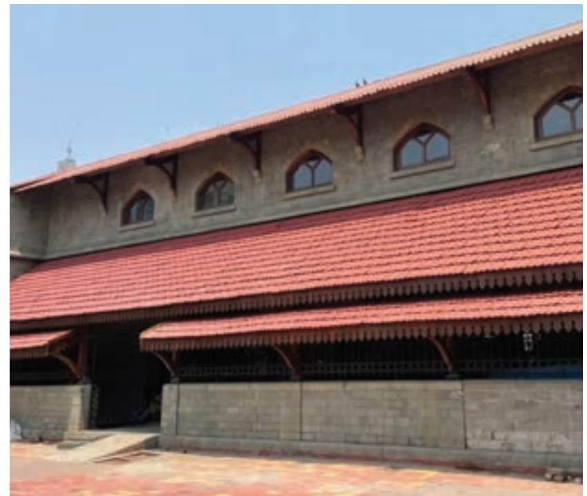
Exterior Façade- After Restoration
