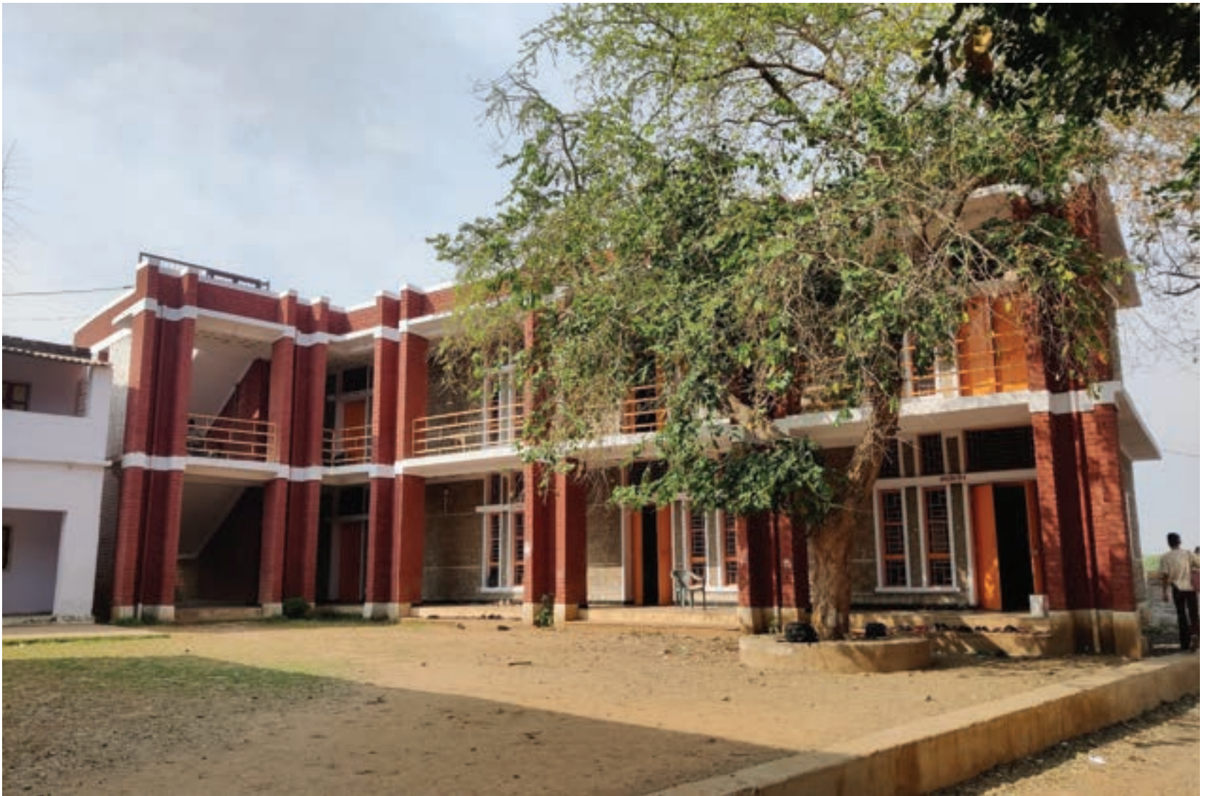
South Façade of the School
