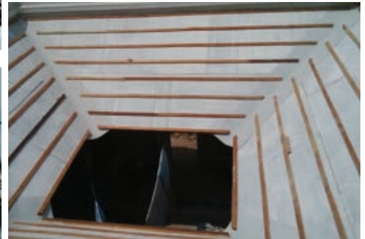
East side courtyard during restoration
