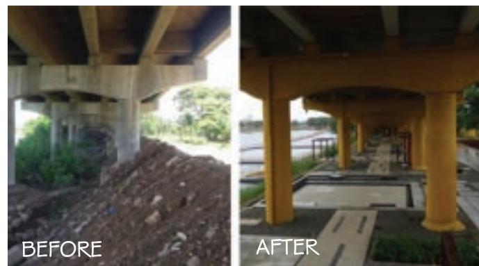
UNDERFLYOVER AT VALANKULAM LAKE
