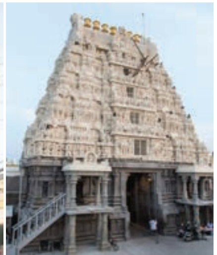
EAST RAJAGOPALAPURAM POST RESTORATION
