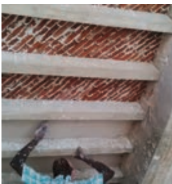
Madras terrace roof during restoration
