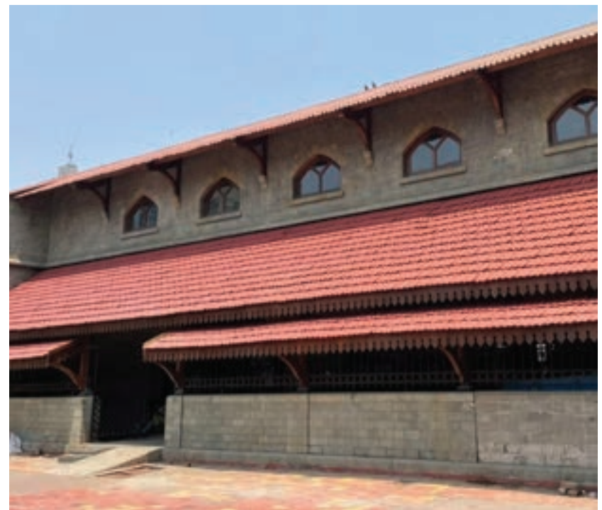
Exterior Façade- After Restoration
