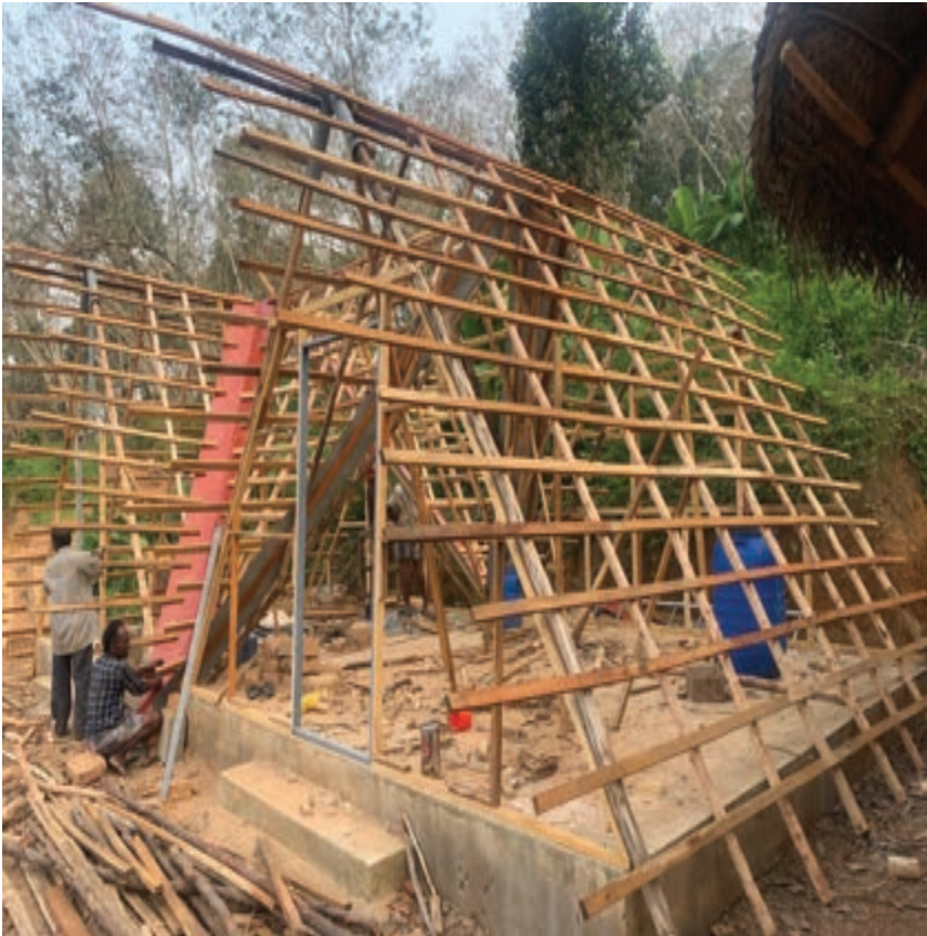
Photos during construction
