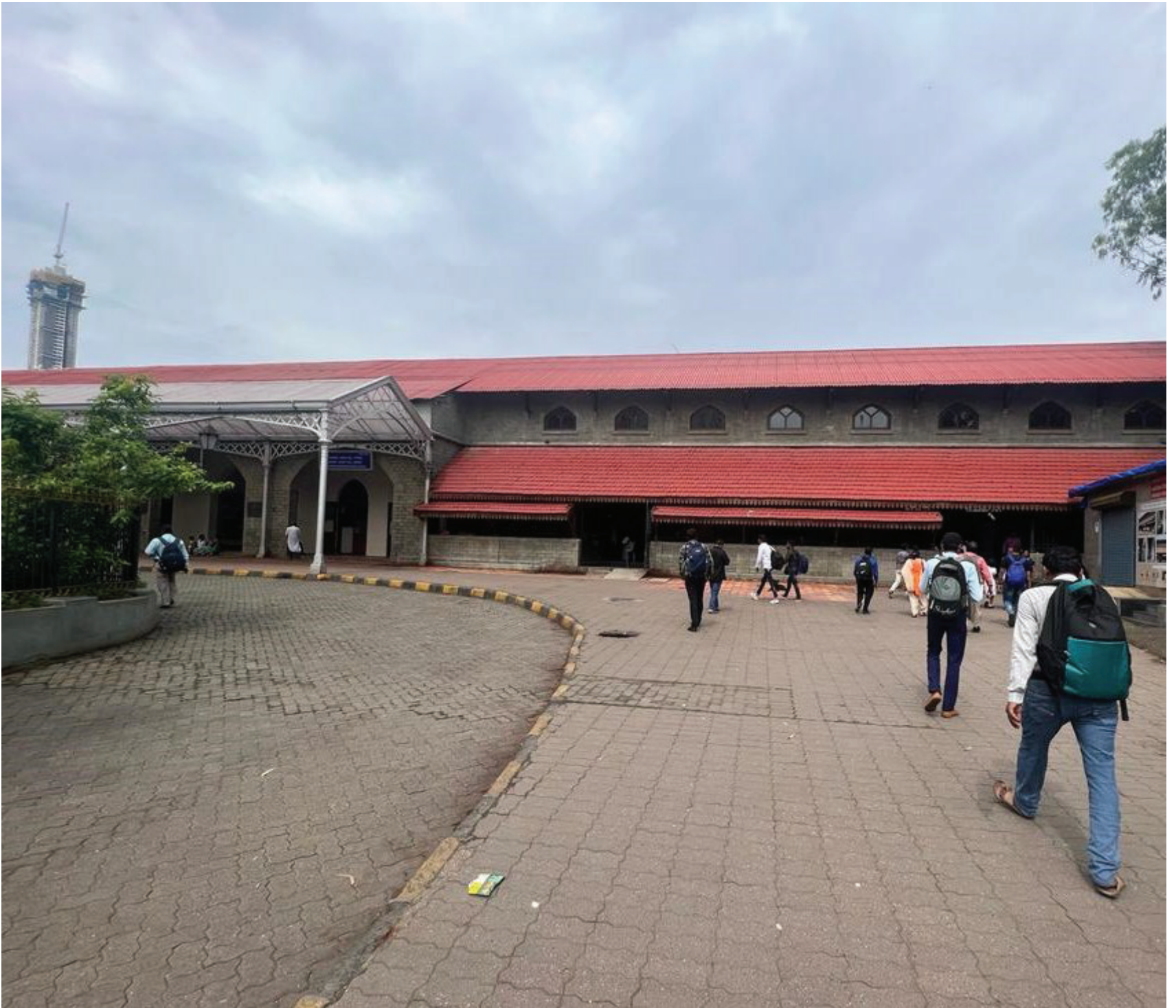
Exterior façade of the station building after restoration with original Gothic details
