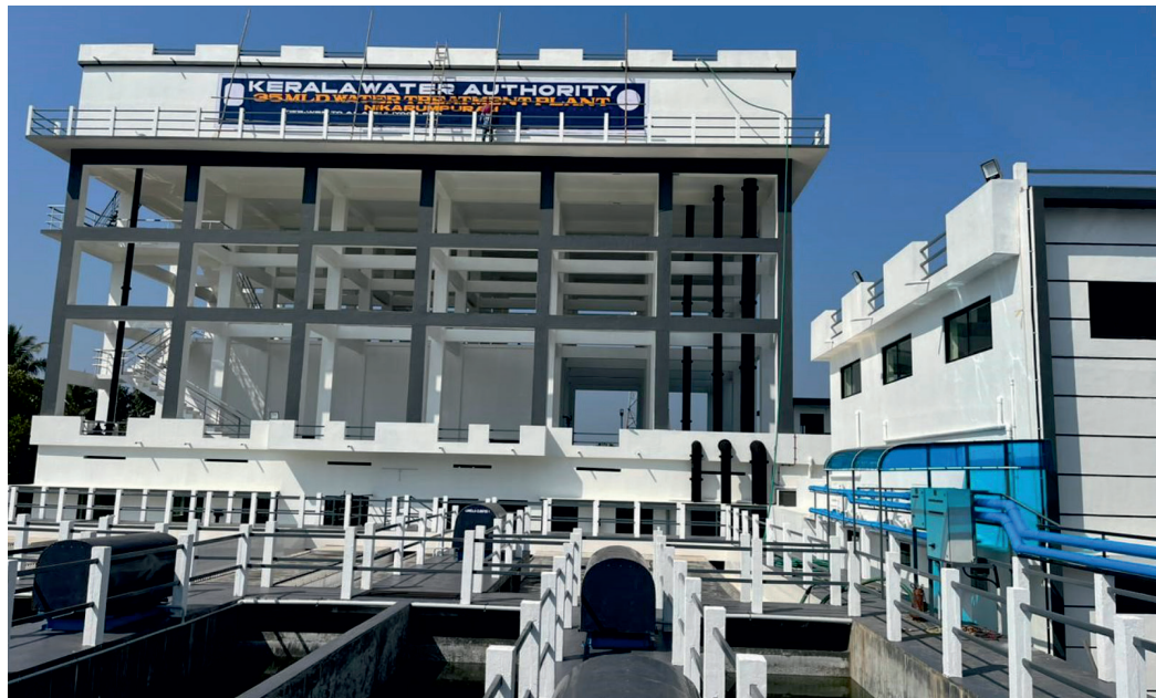
Water Treatment Plant at Chengannur Municipality, Kerala
