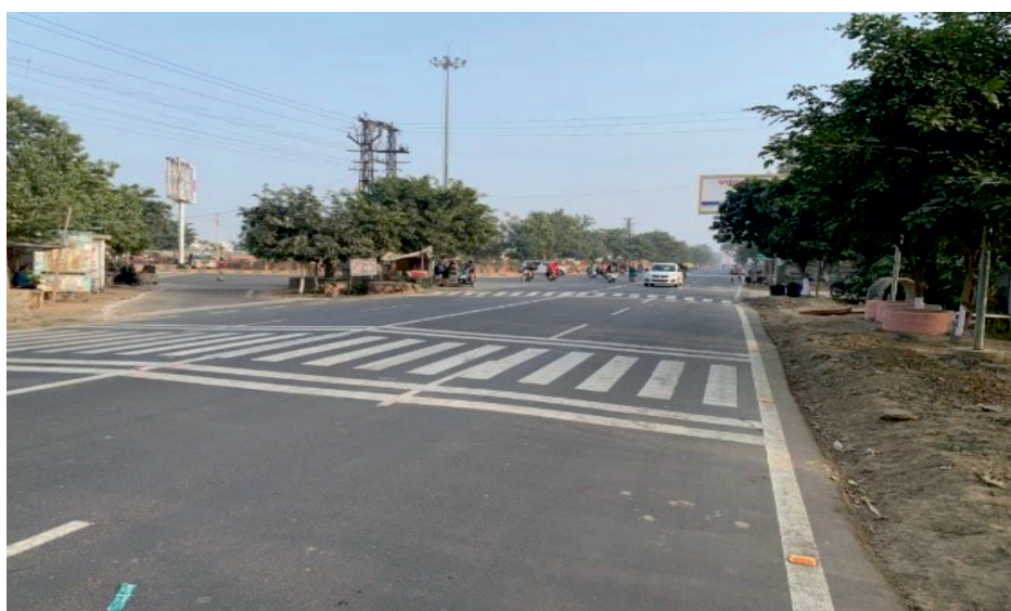
Road restoration and repair works Udaipur, Rajasthan.
