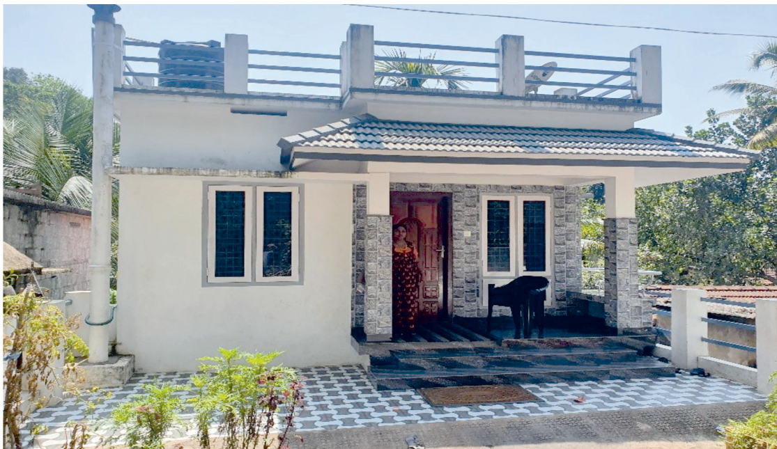
Construction of Houses for EWS (Urban), Kerala
