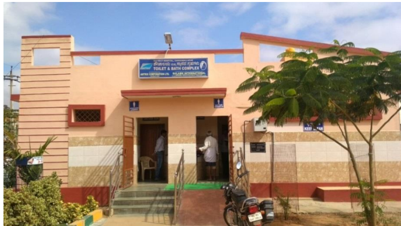
Picture 3: Front view of Community toilets at New Hospital complex, Chikkabalapura
