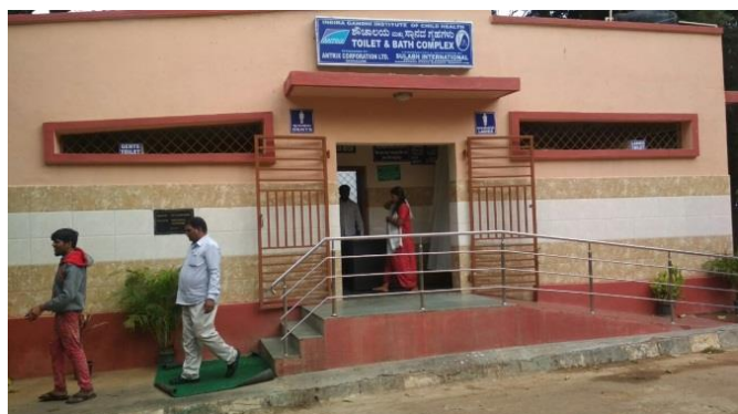
Picture 16: Interaction with end users and front view of community toilet at Bangalore
