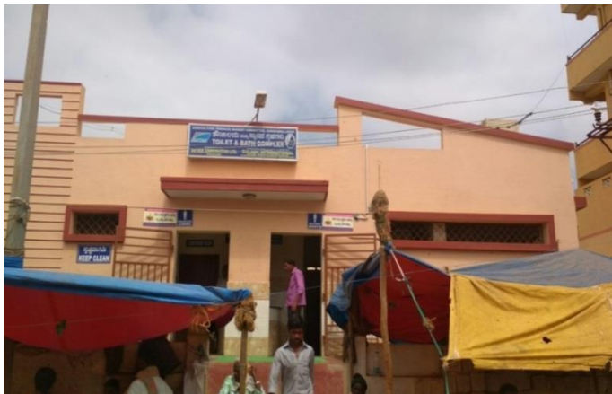
Picture 8: Front view of Community toilets at Chikkabalapura APMC
